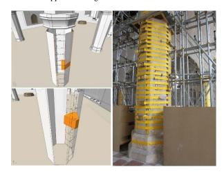
Figure 11. 3D representation of the stone ashlars of the columns, surveyed using both laser scanner and direct instruments.
