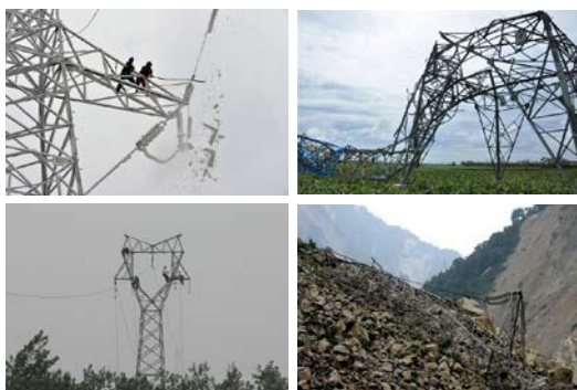
Figure 2 Power line damages brought by extreme weather
