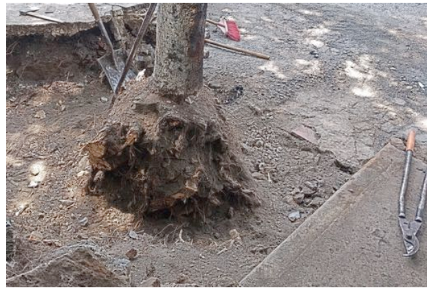
Figure 3. Root mutilated from maintenance works performed from a non-specialized informal contractor. Principal roots were cut and root anchoring lost as the specimen, Liquidambar styraciflua or Sweetgum, develops surface or lateral roots and "severing one major root ... may kill up to 25 percent of the tree root system" (Shamoon, 2012). The tree was removed next day due to severe instability.
