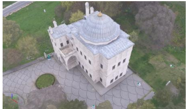
Figure 5. The generated 3D point cloud of the study area
